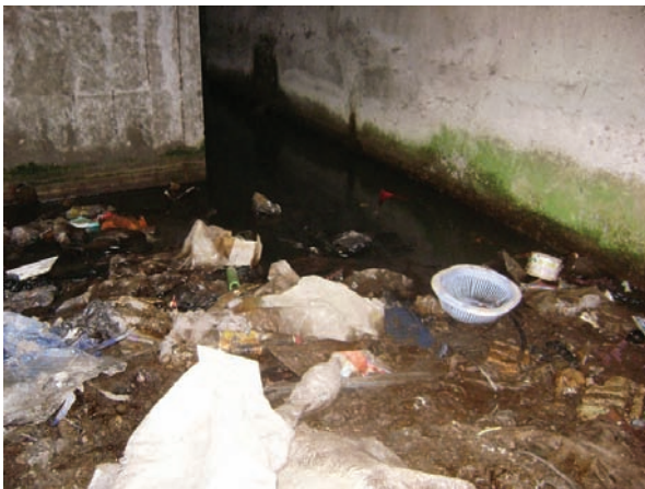
Picture 7: Basement of the House #210 in Senaki Military Settlement
